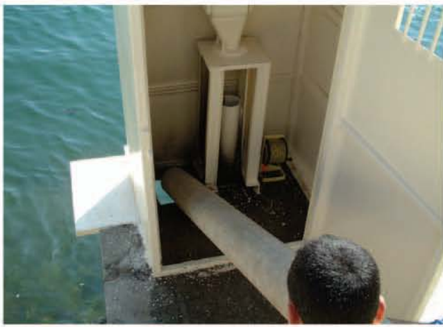
Figure 6: Installation du tube en ethernit
